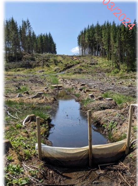
Silt traps in a forest managed by Veon.
